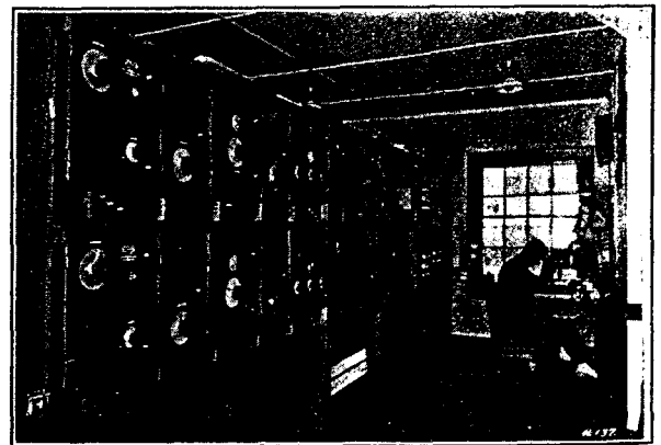
FIG. 25—SHIELDED RECEIVING SETS, RIVERHEAD, LONG ISLAND
